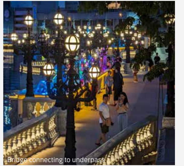
Bridge connecting to underpass
