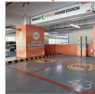
Installed the first electric vehicle charging stations in Bonifacio Global City
