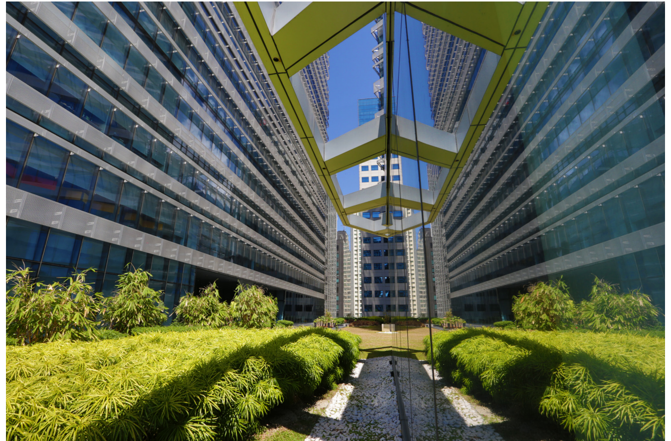
The Sky Park on the 8th level of Six/NEO and Seven/NEO feature native plants and shrubs that contribute to the cooling of the building.
