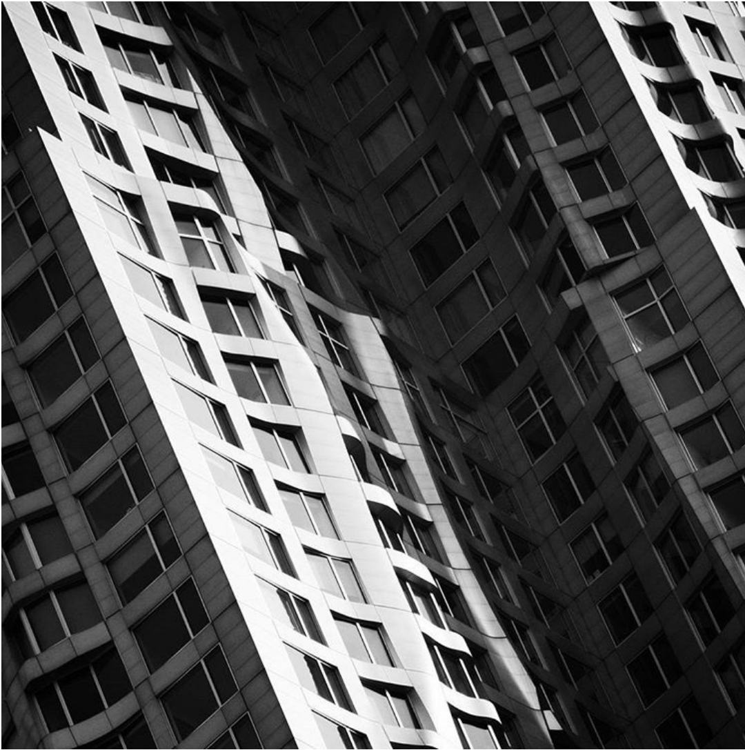
8 Spruce Street by Frank Gehry, New York City, USA
